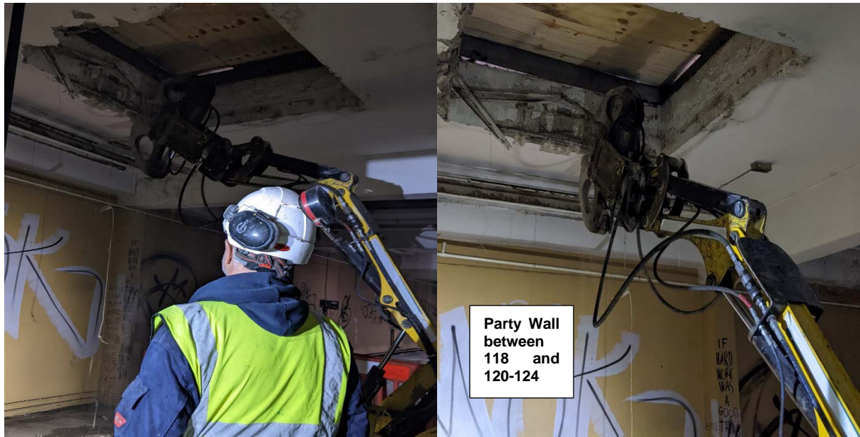
A4.9: Brokk 90 – Slab breaking, First Floor Roof
