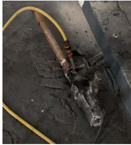
A4.2: Column Coring
