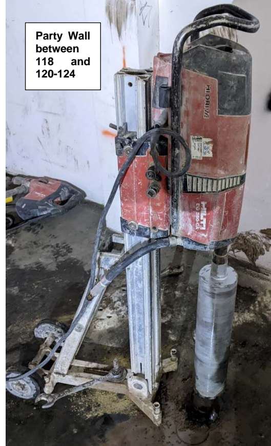
A4.8: Stich (core) Drilling – First Floor
